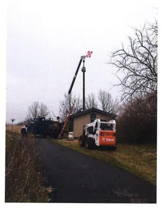
Prairie Landing replaced the motors, shafts, and pumps at the course irrigation pump station. The pump station supplies and charges the irrigation system. The motors, shafts, and pumps replaced were the original units that were installed when the golf course was constructed more than 25 years ago.
