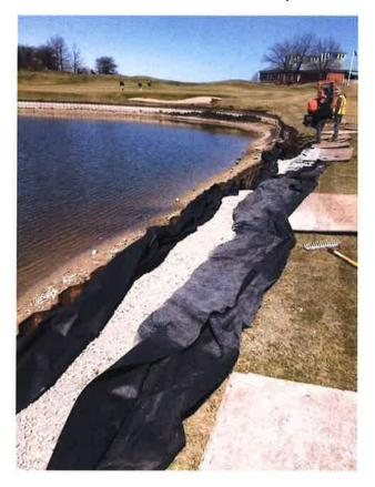
Prairie Landing completed pond abutment and seawall erosion repairs near Holes #9 and #18. Soil erosion between the fairway and the seawall caused an unsafe void that had to be restored to its original condition. The repair included installing a geotextile fabric liner, backfill with stone and restoration to its intended grade.
