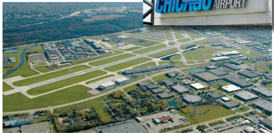
Some 300 aircraft are based on the field and approximately 200,000 take-offs and landings occur annually at Chicago Executive Airport.
