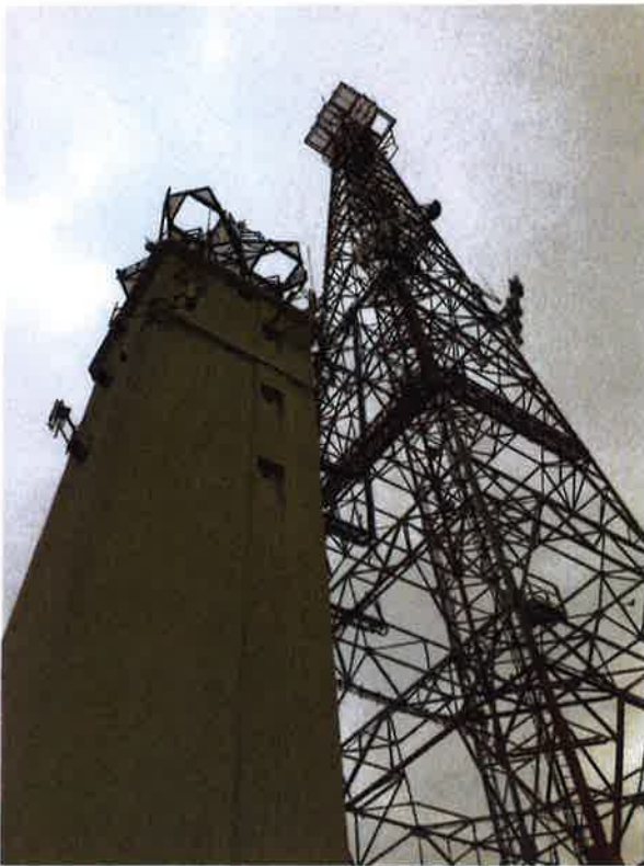
Building 170A High Rise Tower 170 Wall Street – Glendale Heights, IL
