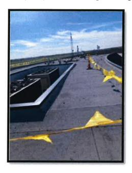
The Airport Authority completed roofing improvements at the DuPage Flight Center, Government Center, and SE Ramp Hangar. The improvements included replacing EPDM roof membranes, fluid membrane application, insulation replacement, flashing repairs, and mansard roof panel replacement.
