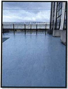
The Airport Authority completed a project to replace the existing epoxy surfacing on the 20,000 SF exterior Flight Center cantilever deck. In addition, decorative vertical security fencing was added to the north and south areas of the deck.
